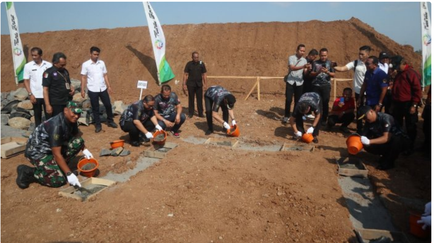
(Foto istimewa) Ground Breaking Lapangan Tembak Pura Group
